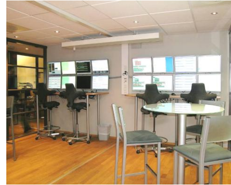
Network Control Center (NCC)
